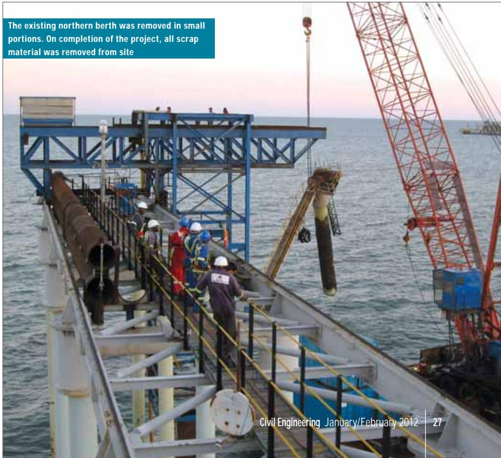
The existing northern berth was removed in small portions. On completion of the project, all scrap material was removed from site
