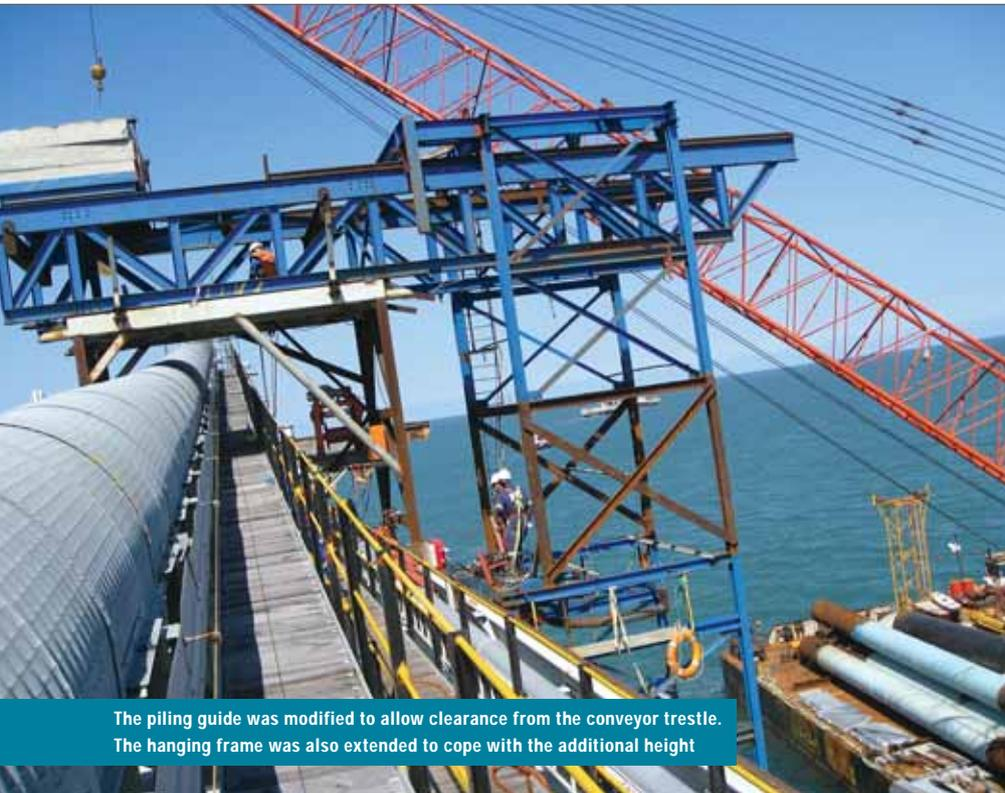
The piling guide was modified to allow clearance from the conveyor trestle. The hanging frame was also extended to cope with the additional height
