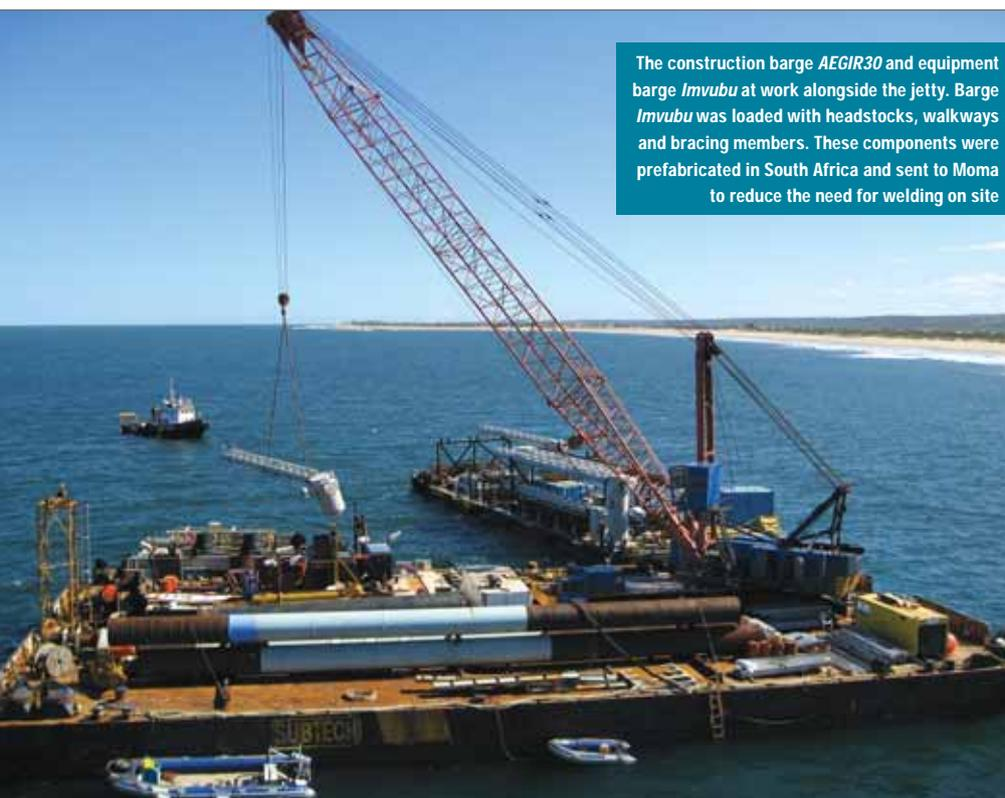
The construction barge *AEGIR30* and equipment barge *Imvubu* at work alongside the jetty. Barge *Imvubu* was loaded with headstocks, walkways and bracing members. These components were prefabricated in South Africa and sent to Moma to reduce the need for welding on site
