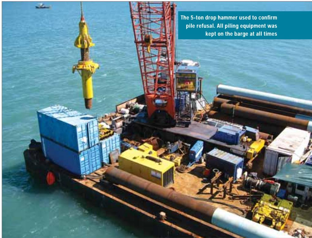
The 5-ton drop hammer used to confirm pile refusal. All piling equipment was kept on the barge at all times
