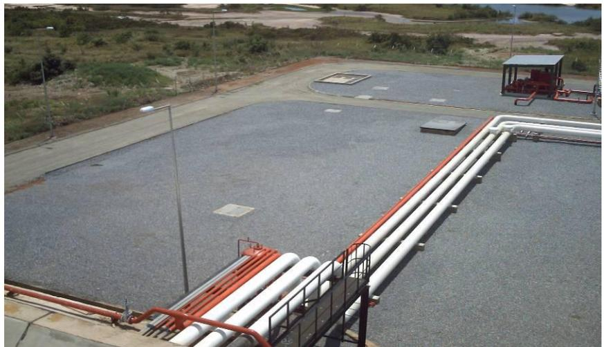
The imported 150mm of sub base material was compacted to 95% MOD AASHTO density. Kerb stones were then laid, followed by the 150mm crushed G4 Grade base course material. The base course material was then mixed, placed and compacted to the required specification, 98% MOD AASHTO Density. Sand replacement tests were carried out to ensure compaction requirements. Survey control was also employed during all the construction stages to ensure all required slopes and cross falls were attained.
