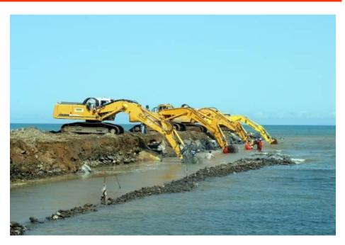
Within a month of the award, PMI successfully lowered the pipeline by more than two meters, guaranteeing the required natural cover through the surf zone.
