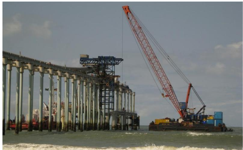
Onsite preparation work started in February 2011 and Construction works commenced in the beginning of March after the arrival of the barge and piling equipment.
